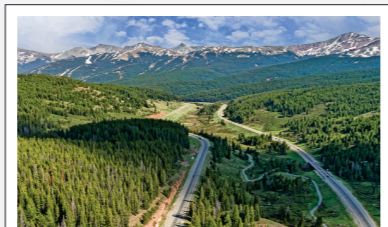
Highest section of the freeway at 3,250m. Just 999 miles to go
